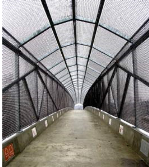
Fairfield Loop Trail Bridge in Iowa
